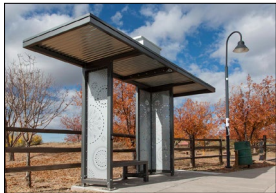
Meridian Contracting / Santa Fe NM
